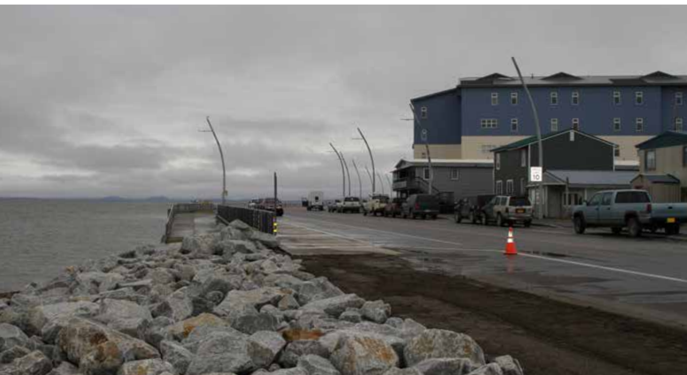
Rapid coastal erosion is one of the many impacts of climate change in the Arctic that damage infrastructure. In Kotzebue, Alaska, Shore Avenue was rebuilt because erosion had reduced it to less than two lanes and was forcing traffic onto adjacent property.
